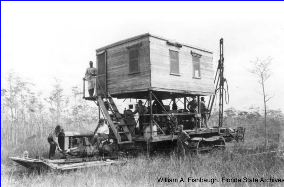
Drill rig used for Tamiami Trail construction, late 1920's
